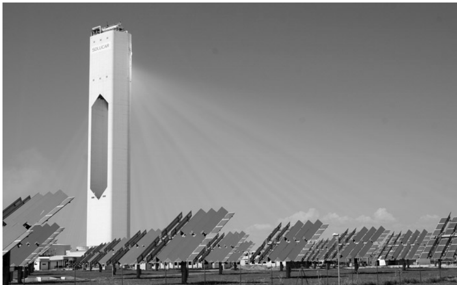
Figure 3.11 Concentrated Solar Power Tower – Solucar, Spain Project.
